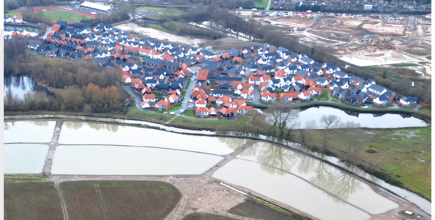
↑ Aerial view of the new wetland scheme at our development in Conningbrook, Kent.
